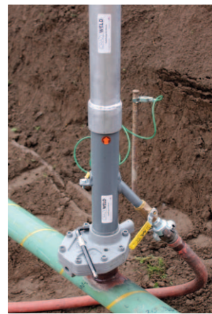
Above: Air mover in use with gate valve
