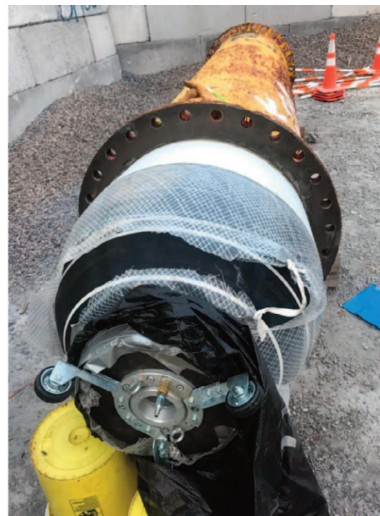
The inflatable "bladder" designed to inflate inside the pipe segment, ensuring that the adhesive liner was flush with the pipe
