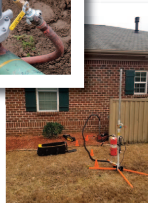
Above: Air mover in use with gate valve
