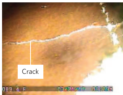
Figure 9. CI Circumferential crack
