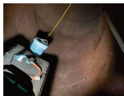
Figure 19. Curtain grouting injection ports
