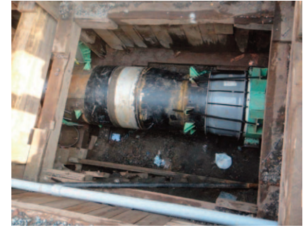
Figure 30. Actual guide pipe field installation with reducer at 30-inch inlet
