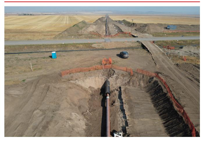
Figure 3. If a road can't be closed, why not go under it? Having straight open workspace to accommodate a single pull section is increasingly rare
