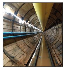
Figure 3. Tunnel support system was steel ribs and wood lagging. Rib expander was utilized
