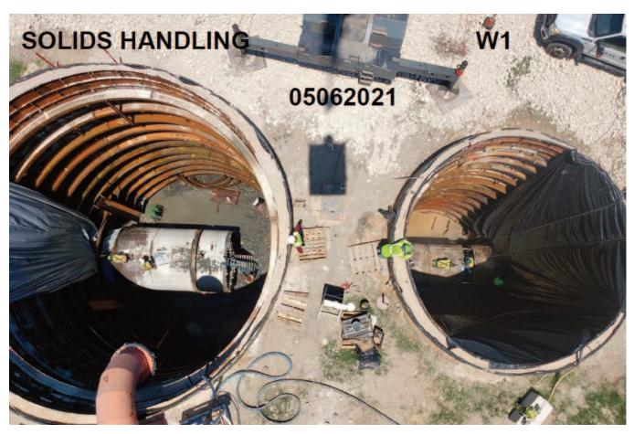
Figure 8. Dual Tunnel TBM Hole Throughs on Adjacent Shafts - Same Day (Image courtesy of SAK. Used with permission)
