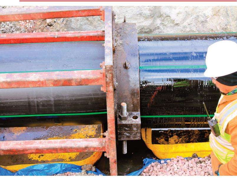
The new 36-inch HDPE pipe replaces the corroded ductile iron pipe (Photo credit: Murphy Pipeline)
