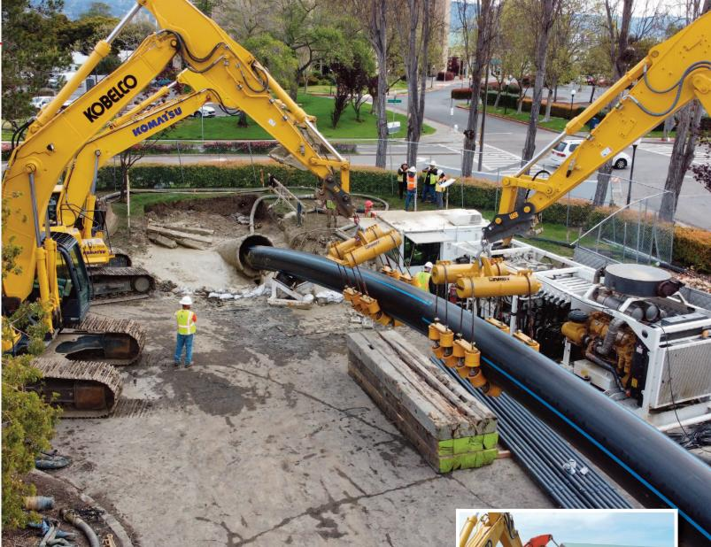
Figure 1. Steel, HDPE and FPVC pipe all elastically bend to adhere to above-ground curvture
