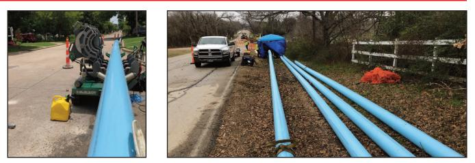
Joint fusing and pipe staging area. Sticks of PVC are joined to full run length prior to the day of the burst, stored conveniently out of the way near the insertion point
