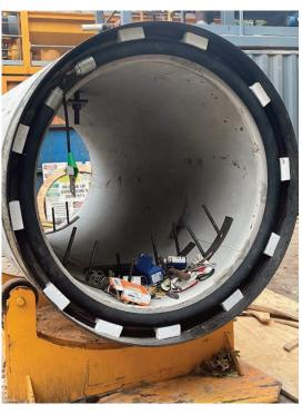
Figure 5. RCP hydraulic joint configuration
