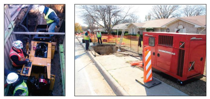
Machine pit dimensions need to be only big enough to accommodate a 4-foot by 12-foot shore box, at a depth not much deeper than the lay of pipe being replaced
