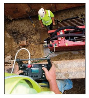
Enhanced safety. Some modern pulling machine designs free the operator from the pit, offering a superior view of the operation and of worksite surroundings during an installation
