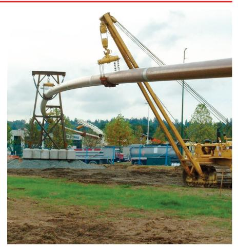
Figure 4. Pullback towering over a road
