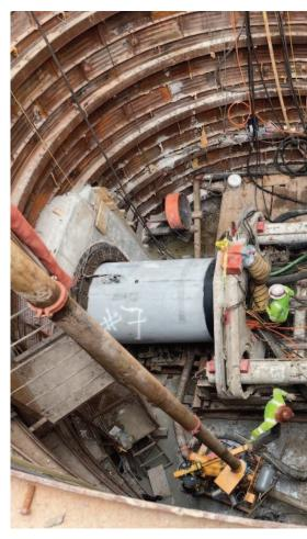
Figure 6. Jacking frame and casing pipe wihin installation shaft
