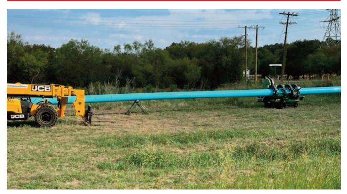
Figure 4. 20-inch fusible PVC pipe
