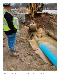
Figure 5. Boring pit showing a high groundwater level
