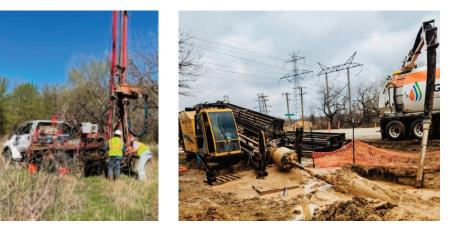
Figure 3. Geotechnical boring rig (left) and Directional boring rig (right)
