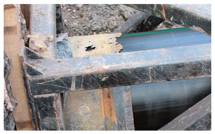
Replacing the corroded ductile iron pipe that had been eaten away by sulfuric acid caused by sewage, the HDPE pipe is inserted into the destroyed pipe using the CompressionFit method from Murphy Pipeline (Photo credit: Murphy Pipeline)
