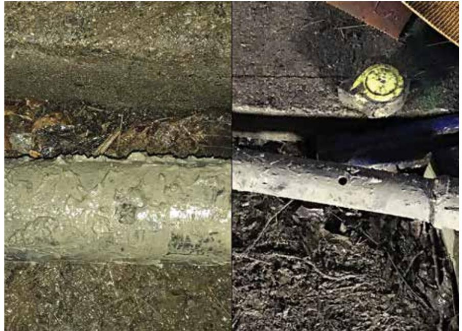
Figure 14. Clogged tremie pipeline before and after cleaning
