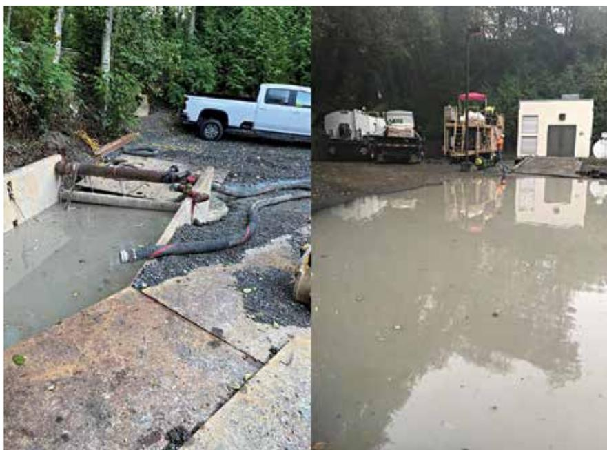
Figure 7. Overflowing drill pit (left) and flooded work area (right)
