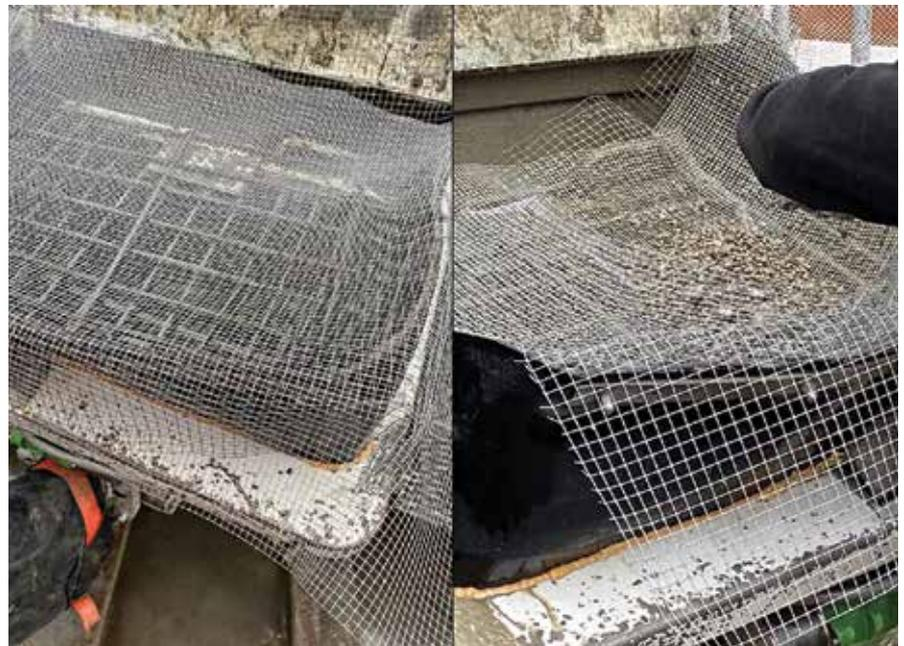
Figure 15. Aggregate captured on screen over grout pump truck hopper
