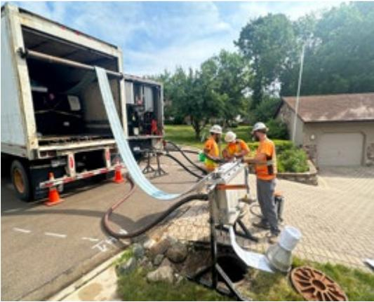
Figure 5. CIPP Liner Installation
