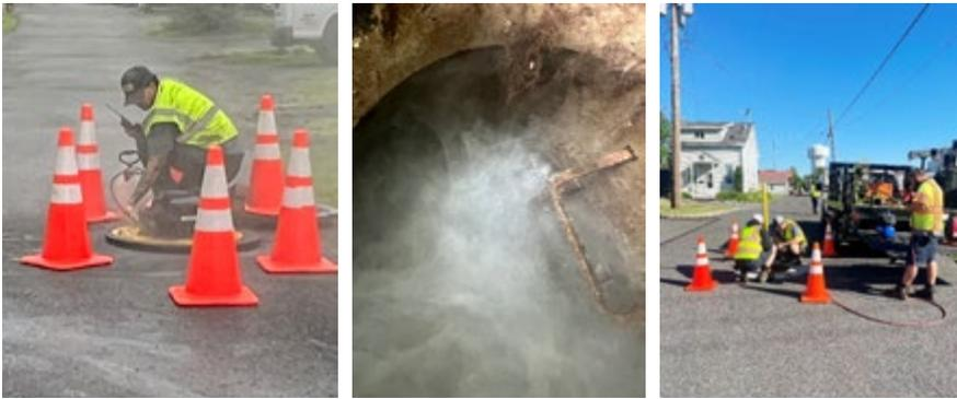
Figure 7. Smoke testing in progress
