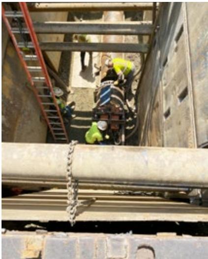
Groundwater control was required during the boring and jacking operation
