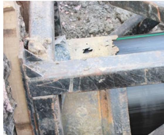
*Replacing the Sioux Falls corroded ductile iron pipe that had been eaten away by sulfuric acid caused by sewage, the HDPE pipe is inserted into the destroyed pipe using the CompressionFit method from Murphy Pipeline
