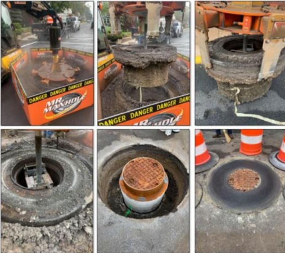
Figure 2. Mr. Manhole Installation System
