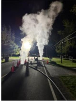
Figure 4. Steam curing CIPP
