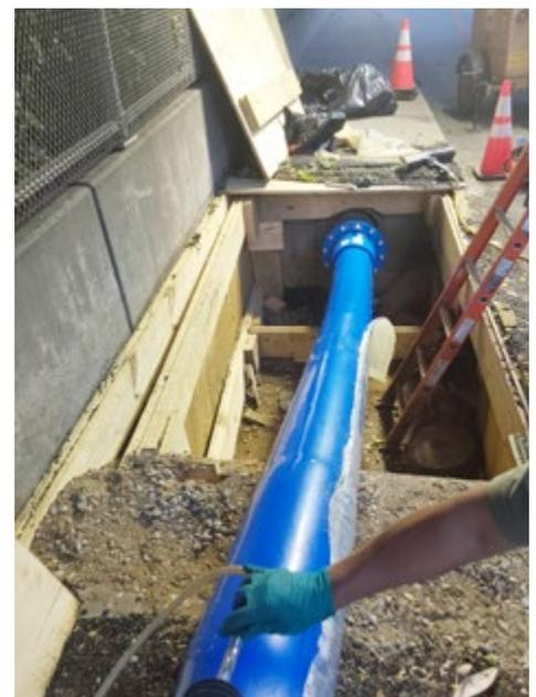
Liner inflation and pressure testing after installation
