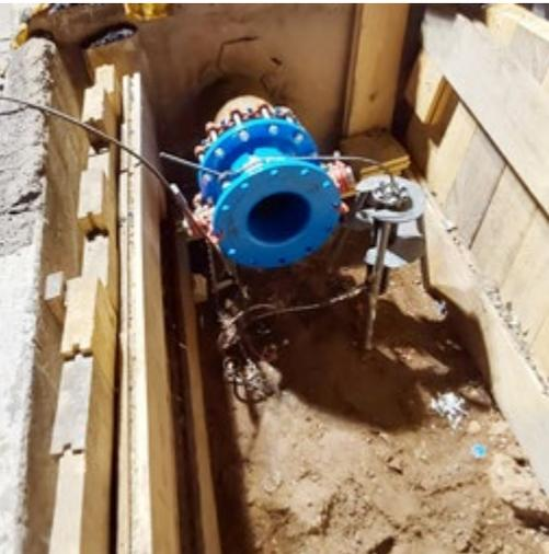
Temporary gate valve installed for pressure testing
