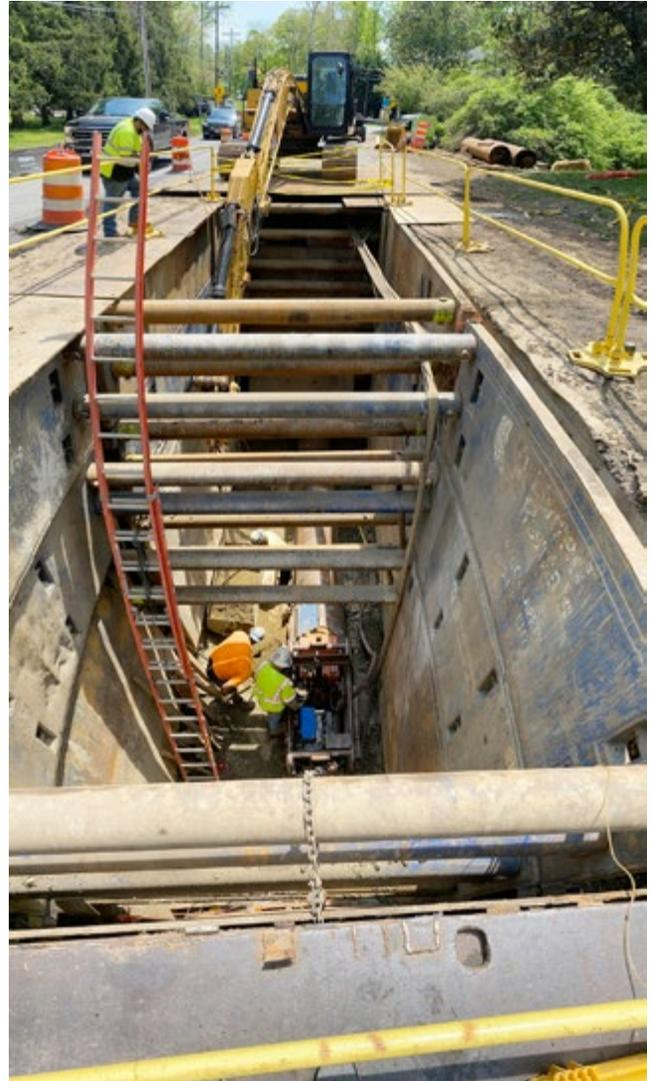
*Safely engineered shoring was important considering the depth of the jacking pit*
