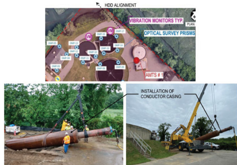
Figure 11. Vibration and Movement Monitoring
