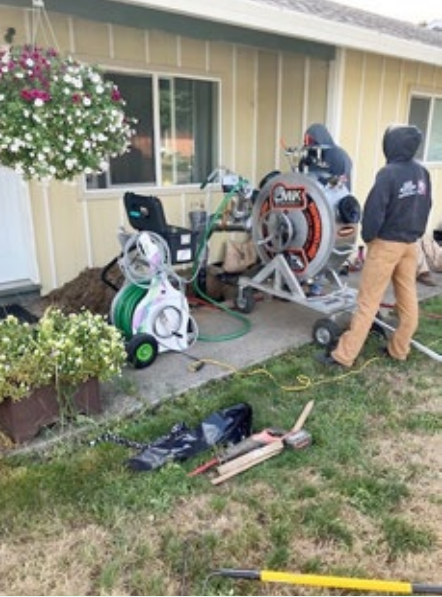
Only one access point is necessary even for longer rehabilitation lengths
