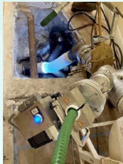
Curing is done immediately after installation of the liner
