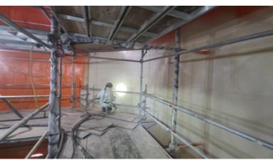
The OBIC system utilizes a structural version of spray foam insulation as a middle layer
