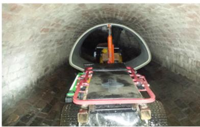
Each GRP segment was maneuvered into place using an electronic motorized cart
