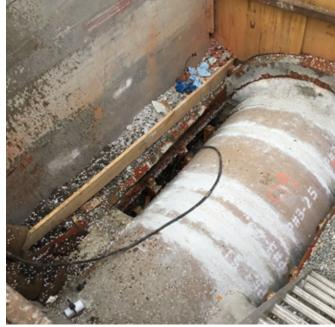
Annular grouting completed the construction process
