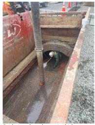
Brick pipes cleaned out using high pressure water, and debris removed by hydrovac
