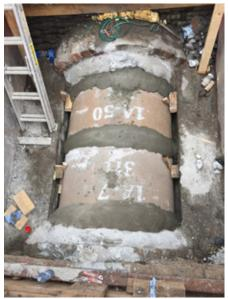
Each seam had internal gasket and external seal
