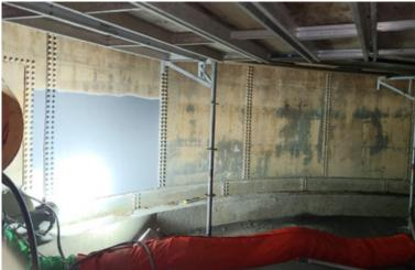
Tanks walls were corroded with serious pitting
