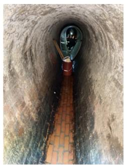
GRP liners conform to the unique shape of the existing pipe
