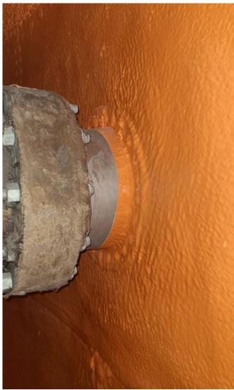
Detail of coating termination against the uncoated utilities
