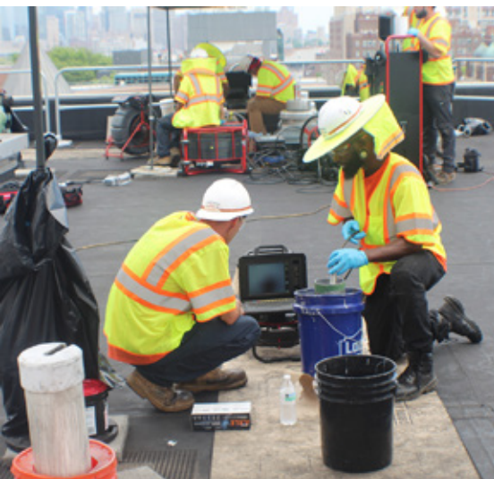
BIPP coating has a two-part epoxy that forms a barrier resistant to corrosion and abrasion
