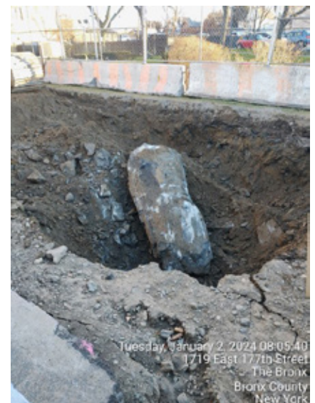
Boulders as large as 10 feet were excavated and removed from the jacking shafts
