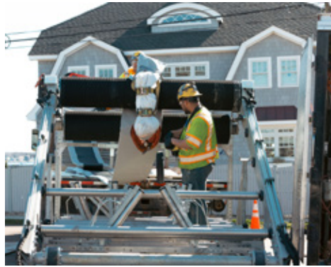
UV CIPP lining is an innovative trenchless process for rehabilitating pressure pipe
