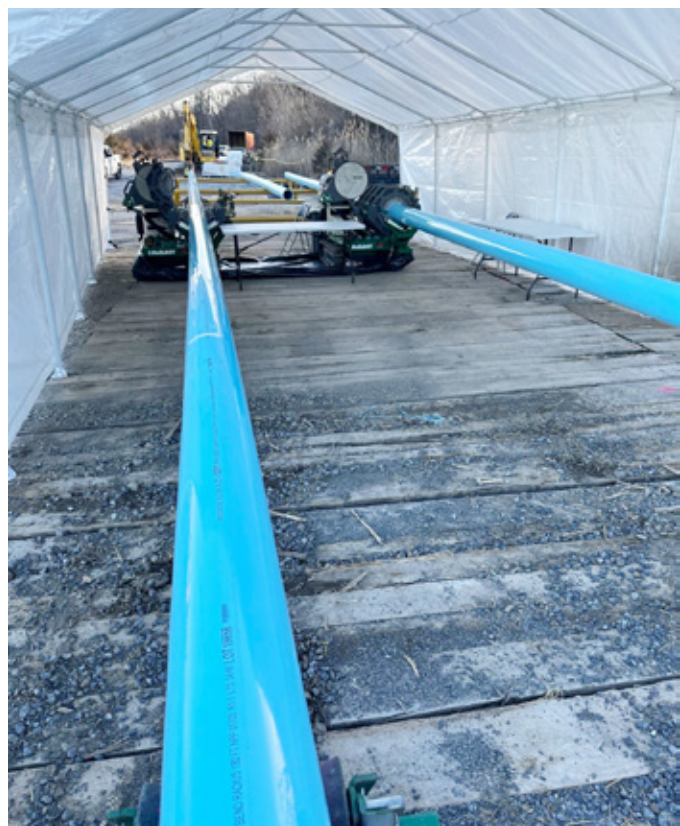
Figure 5: Pipe Fusion Operation
