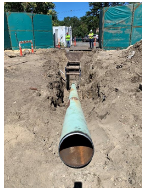
Figure 7: Installation of 16-inch steel surface casing pipe to the top of rock surface and backfill the entry pit
