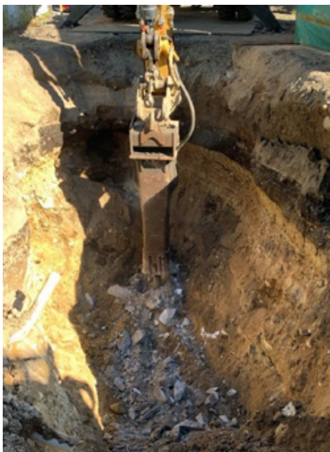
Figure 6: Using hammer to excavate top of bedrock to allow the pilot drill bit to enter the bedrock at the desired entry angle
