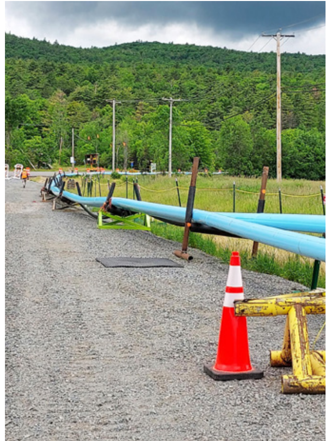
Figure 1: Long Strings of Fusible PVC®
