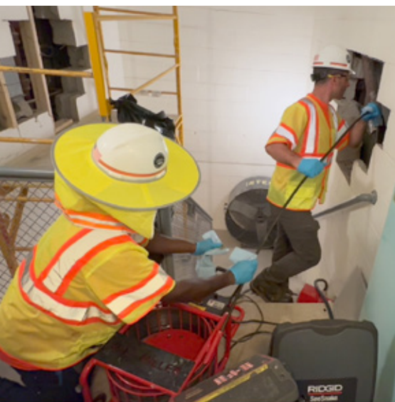
CCTV and cleaning tools are applied prior to BIPP coating
