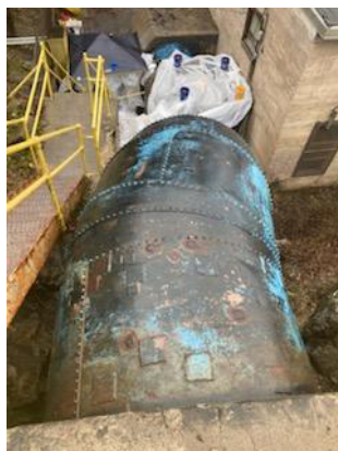
Multiple steel plates had been welded into the structure in attempts to fix the pipe
