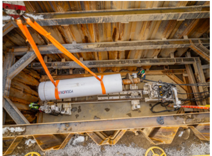
Sending pad 40 feet in length to accommodate both drill and 20-foot casing length segments
