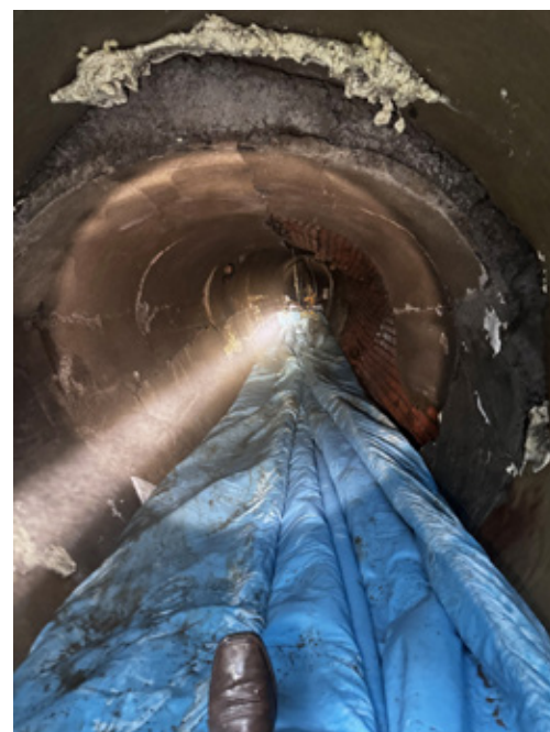
CIPP installation was roughly a 16-hour process from start to finish
