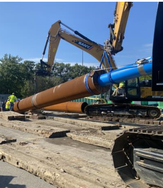
Figure 5: Installation of 48-inch exit casing
