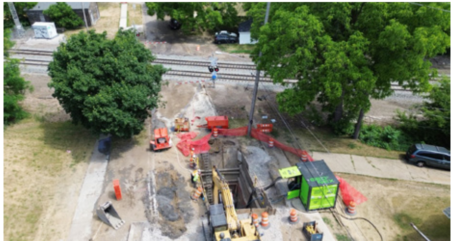
Aerial view of equipment set up to bore under the railway
