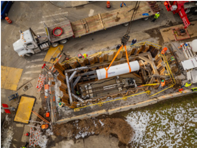
Sending pad 40 feet in length to accommodate both drill and 20-foot casing length segments
