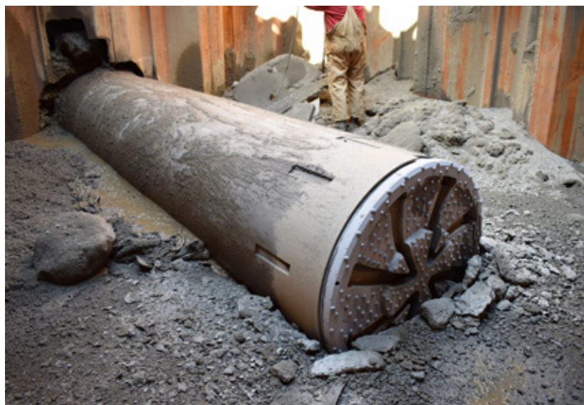
Drilling through obstructions, mixed and varying ground composition took 5 1/2 weeks
