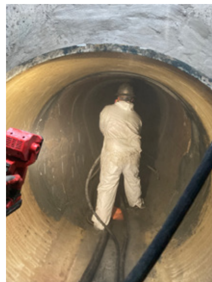
Centrifugally Cast Concrete Pipe (CCCP) lining was done through the delaminated portion
