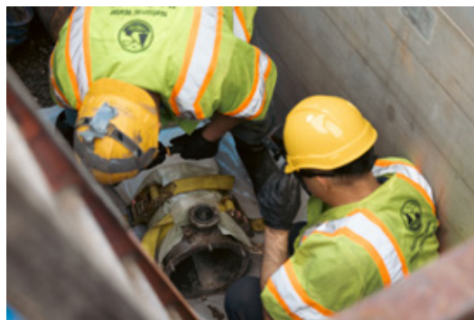
Cured liner forms a new, seamless pipe that extends the life of the existing force main
