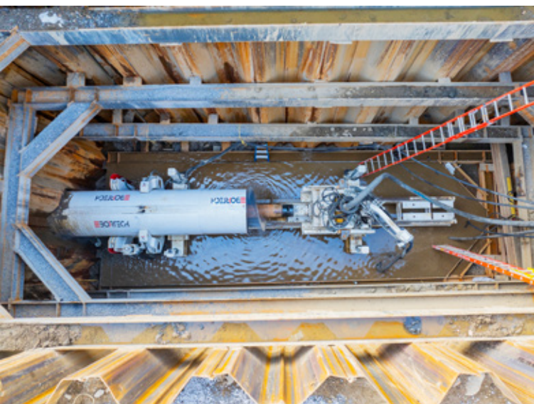
Groundwater penetration added several days to the overall schedule
