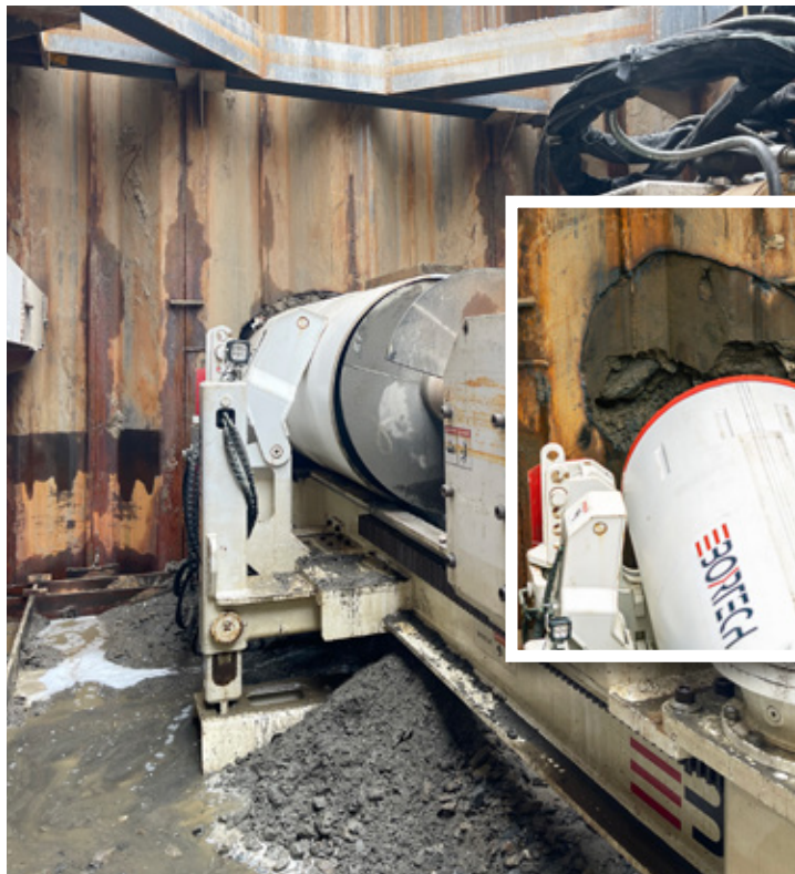
Drill rig advances the casing pipe as required based on formation resistance
