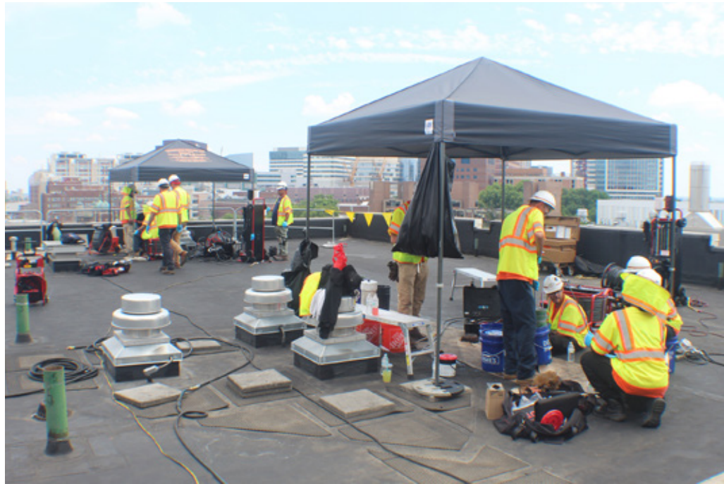
PPM crews apply Brushed-in-Place Coating (BIPP) to vertical roof drains
