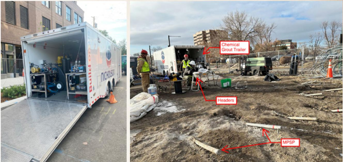
Figure 4: Chemical grout trailer (left); grouting operations (right)
