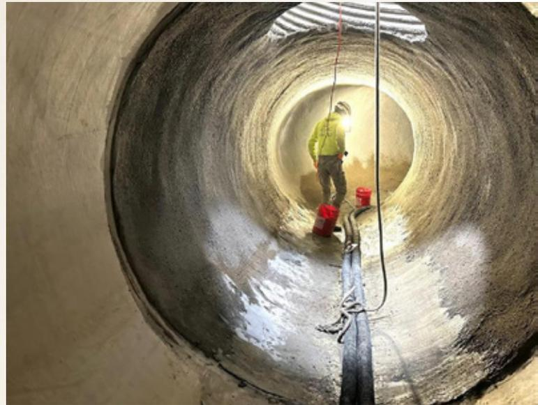
Figure 6: Geopolymer installation in CMP pipeline corrugations (left), completed geopolymer installation through 62-degree bend (right) (Courtesy of Cardinal Coatings)
