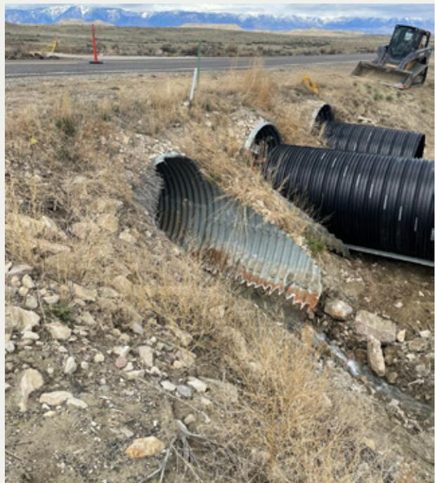
*Contractor adeptly sliplined each section into the existing triple-barrel span*
