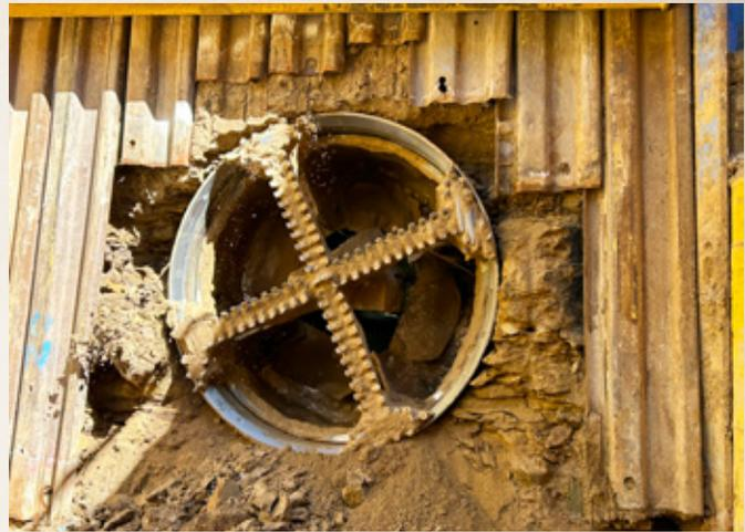
Figure 1: Permeation grouting treatment zone overlay (left); south tunnel within receiving pit (right)
