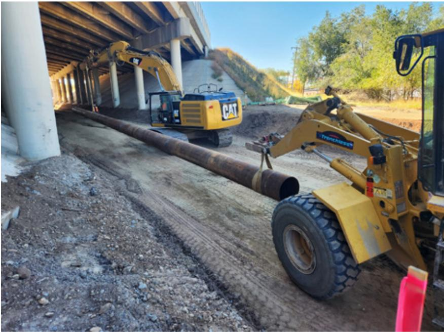
*Open-cut casing installation under a future pedestrian trail*
