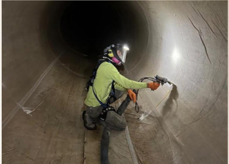
Figure 5: Grout installation ports at diameter transition (left), injection of grout (right) (Courtesy of Cardinal Coatings)
