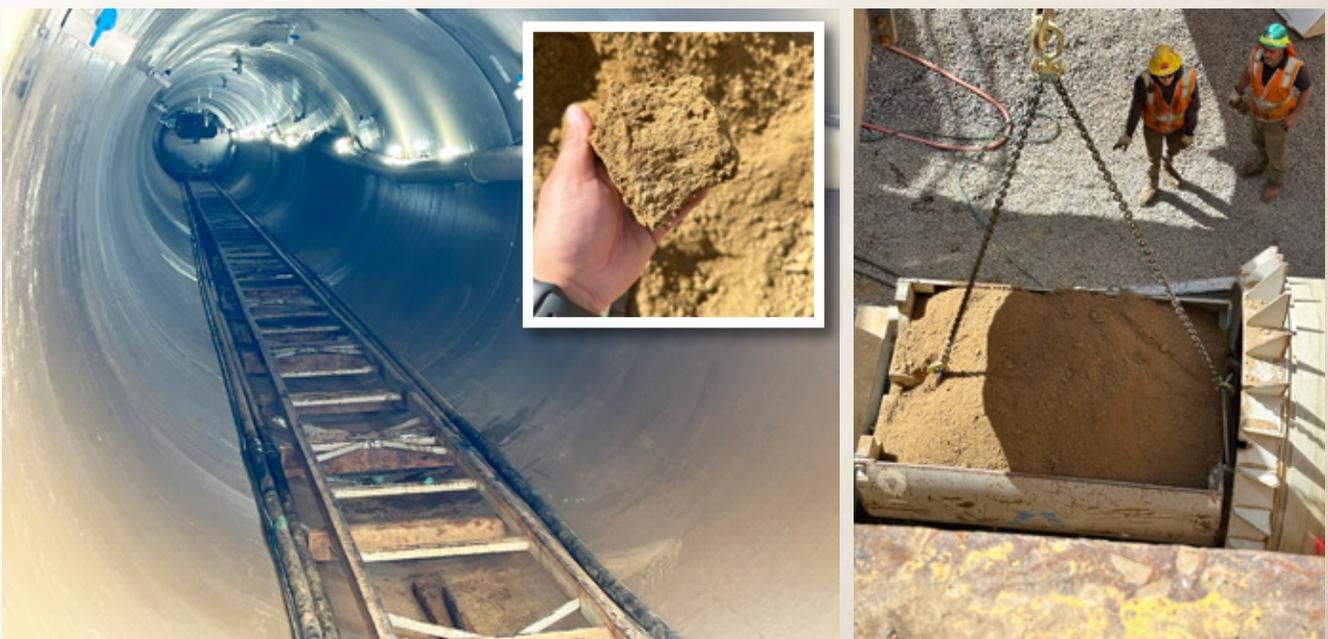
Figure 5: Insite Tunneling Operations (left); Soil Cuttings Bucket (right); Chemical Grouted Silty-Sand (center-top)
