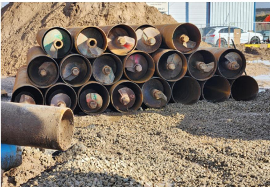
*Auger in casing ready for 365-foot bore*
