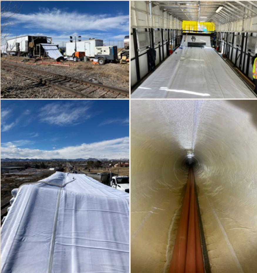
Figure 4: Over-the-hole wetout site layout (upper left), on-site wetout facility (upper right), dry CIPP liner prior to wetout (lower left), finished CIPP liner (lower right)
