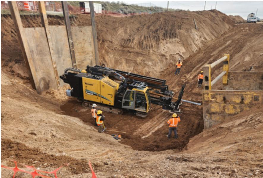
Deep bore pit with ramp for waterline HDD
