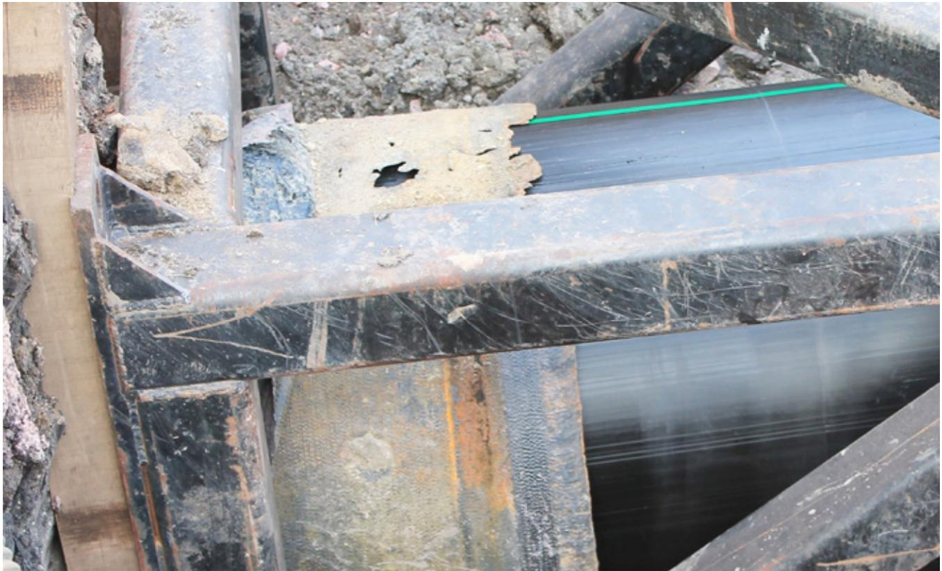
Replacing the Sioux Falls corroded ductile iron pipe that had been eaten away by sulfuric acid caused by sewage, the HDPE pipe is inserted into the destroyed pipe using the CompressionFit method from Murphy Pipeline (PHOTO CREDIT: MURPHY PIPELINE)
