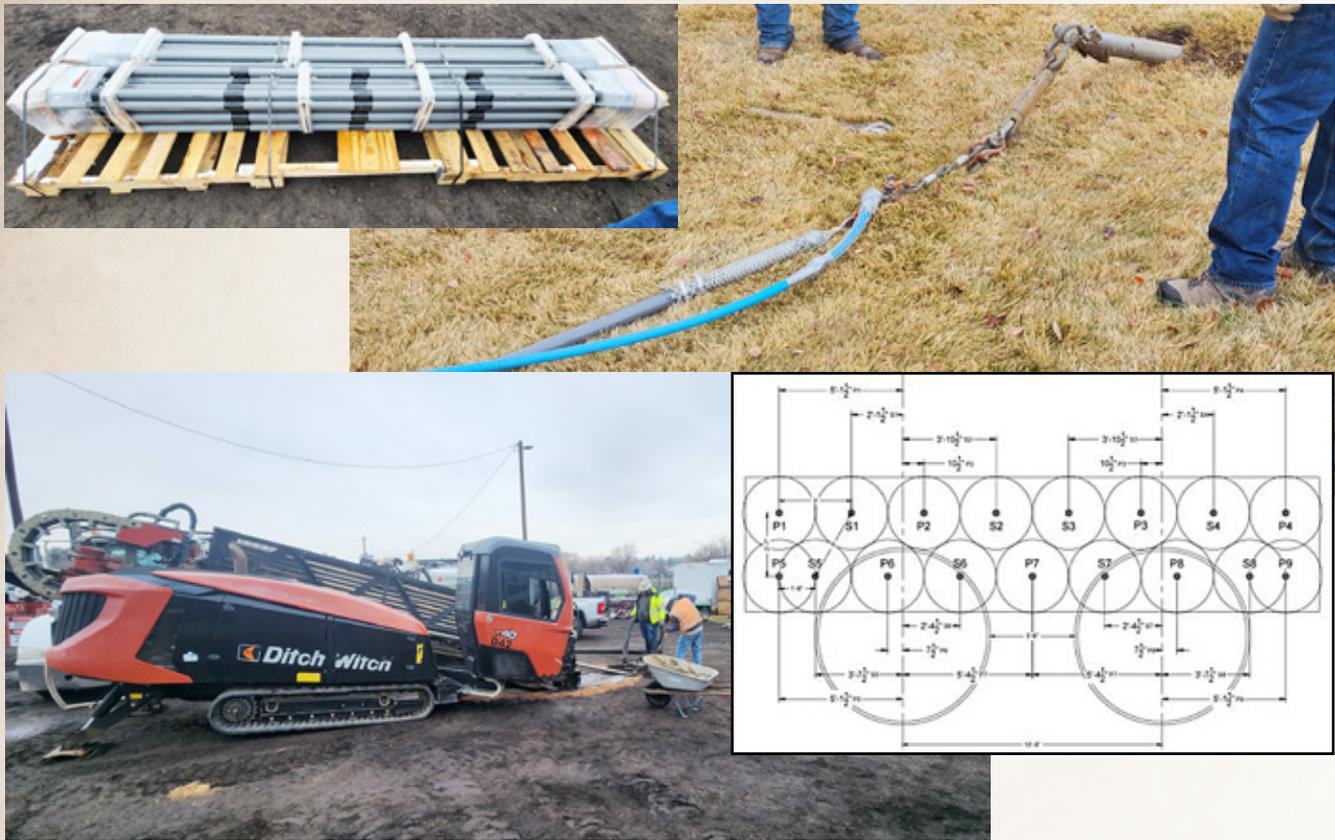
Figure 3: Multi port sleeve pipe (upper left); directional drilling rig (bottom left); connecting MPSP (top right); horizontal hole layout (bottom right)
