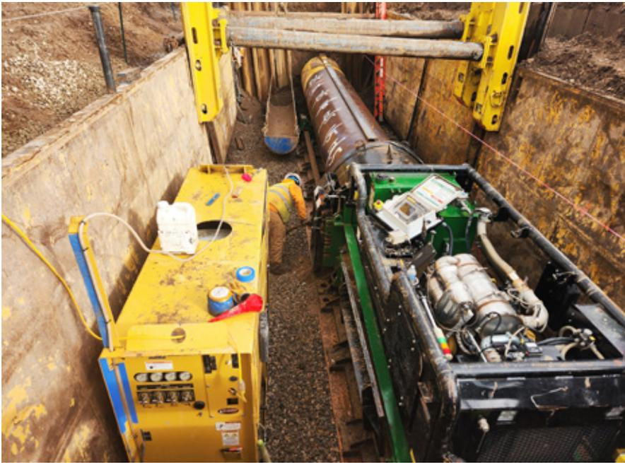
*On Target Steering rig in bore pit with 48-inch casing*
