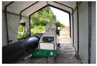
Crews butt-fuse HDPE pipe on a multi-year slip lining project in Saint John, New Brunswick. The city replaced 10 km of 100-year-old cast iron water transmission main by slip lining with new HDPE pipe.
