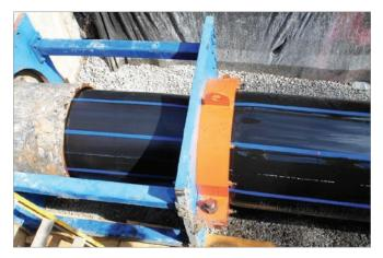
Crews install HDPE pipe with the CompressionFit process to replace a failing water transmission main. The value over slip lining is after the HDPE pipe is pulled in and tension is released, the pipe naturally reverts to form a tight fit within the host pipe. This method maximizes the final internal diameter which allows for greater flow and capacity.
