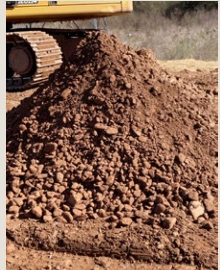
AFTER: A pile of cuttings generated during installation by the horizontal down-hole hammer boring process
