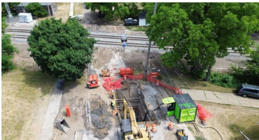
Aerial view of equipment set up to bore under the railway
