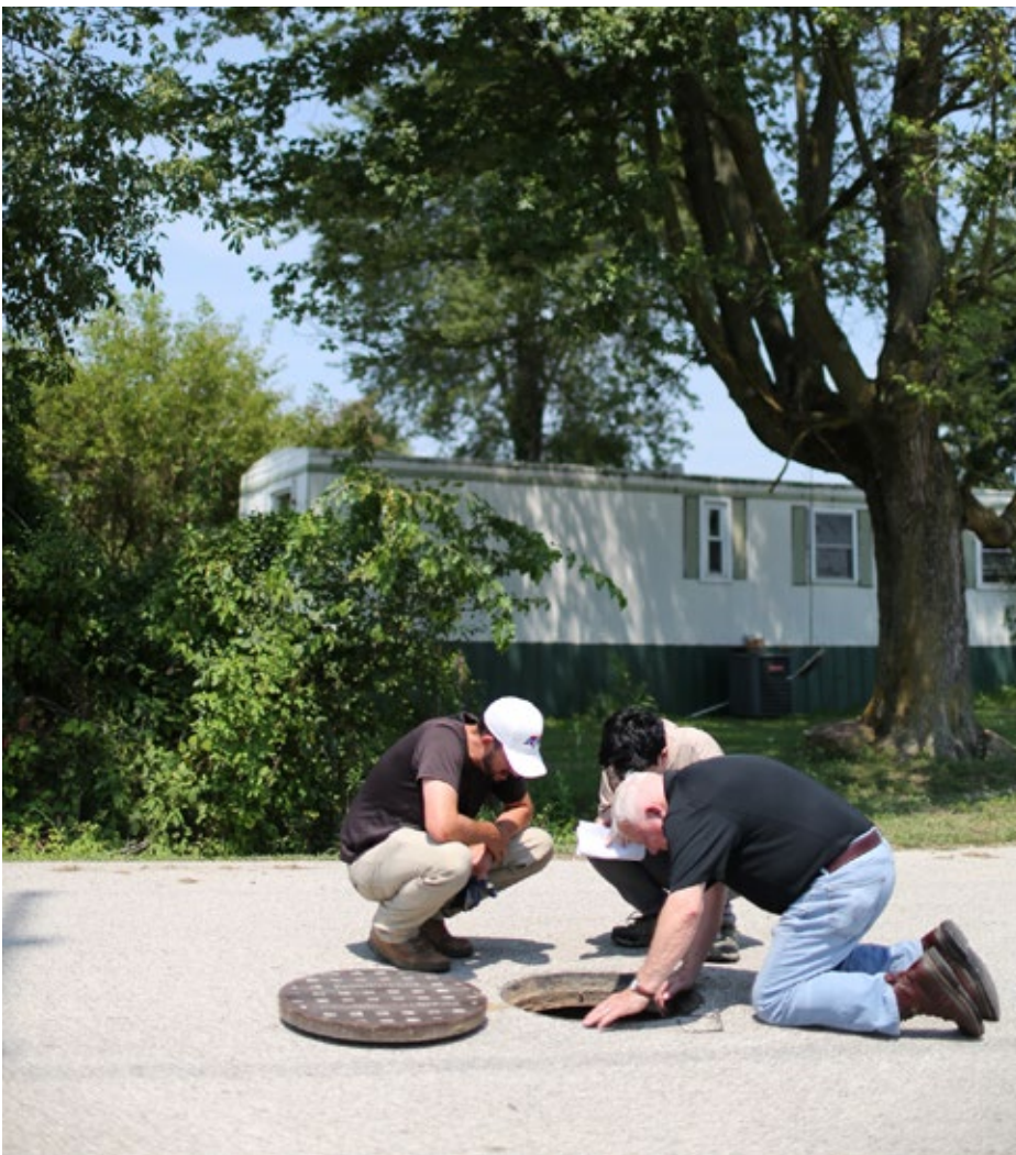
Flow meter location survey in the Switz City wastewater system
