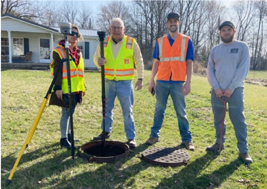
The project team conducted the manhole inspection in Switz City
