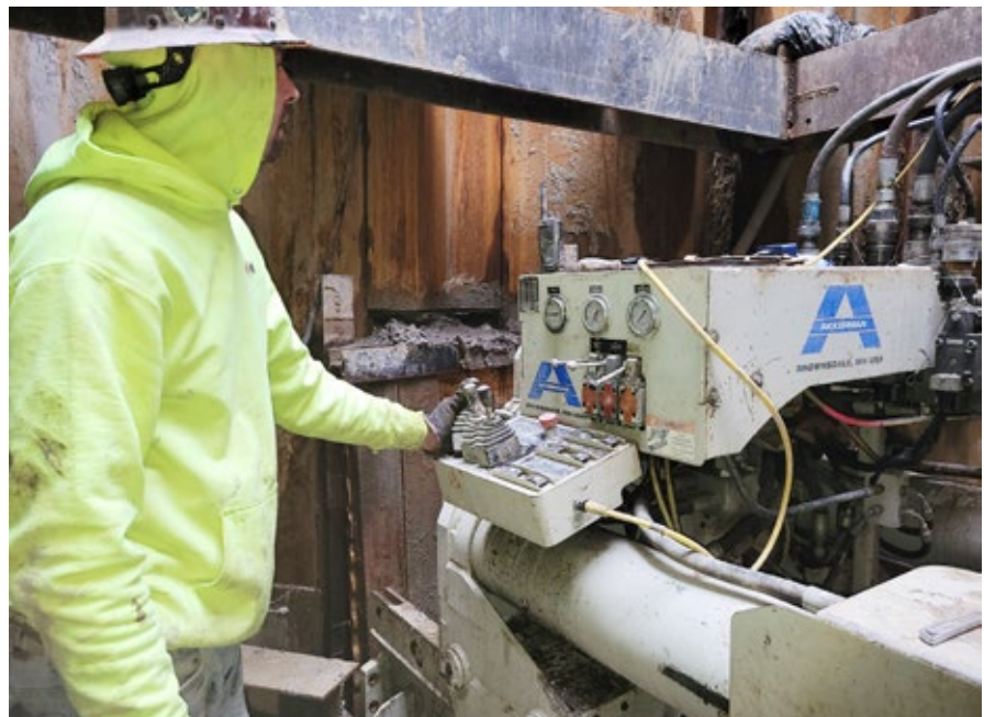
Jacking shaft was a compact 13 feet – one-meter pipe lengths were used for installation
