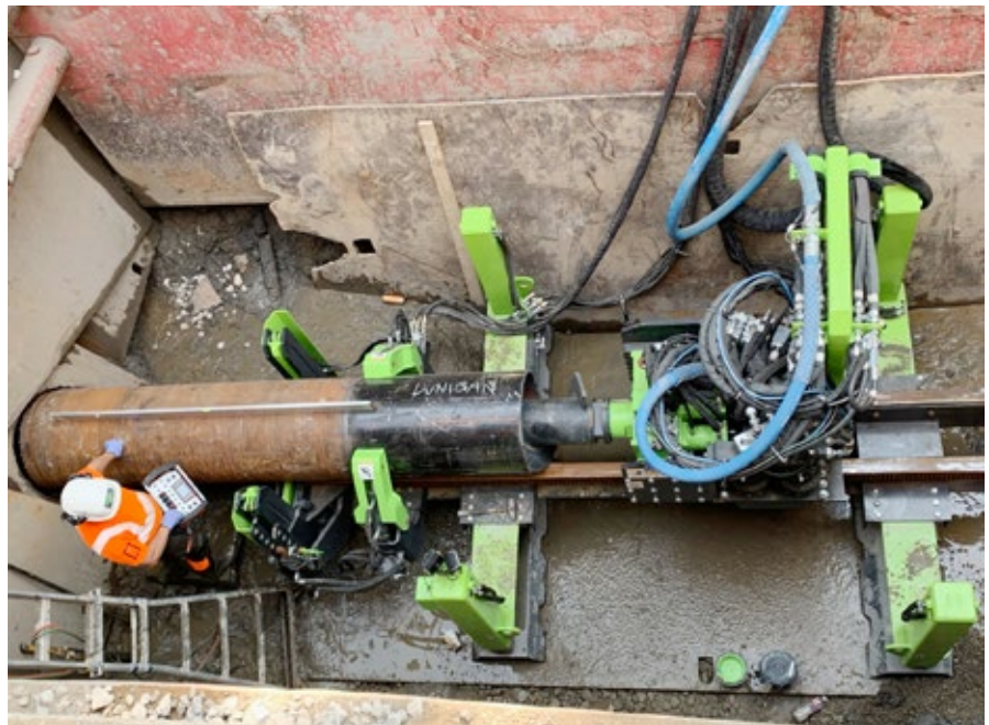
Technician uses the remote control to operate the GEONEX HZR610 drill machine set up for 10-foot casing lengths
