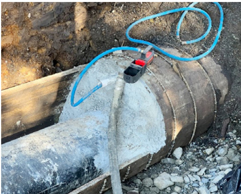
Figure 8. Bulkhead Construction
