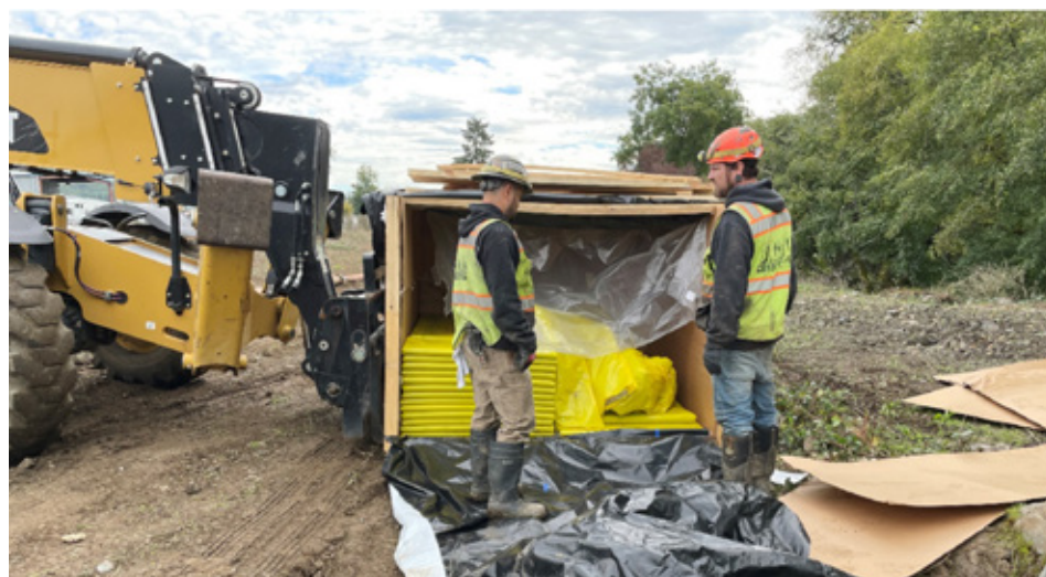
Figure 5. Staged UV-CIPP liner
