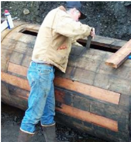
Figure 3. Historical Penstock Repair
