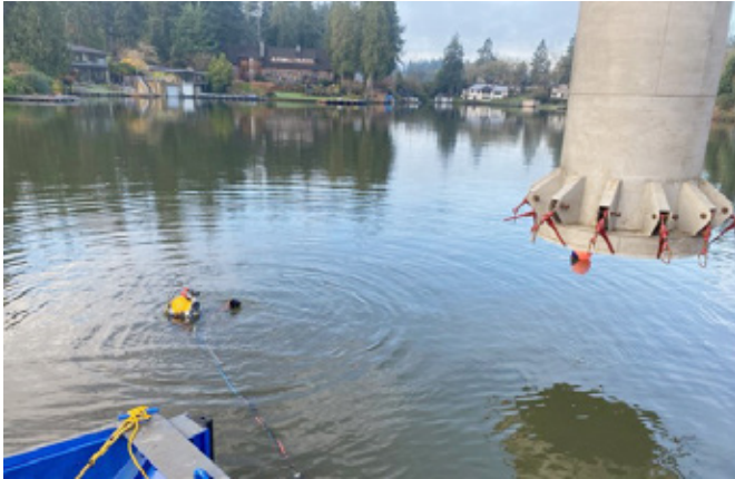
Caissons were installed and dewatered to facilitate access to the sewer
