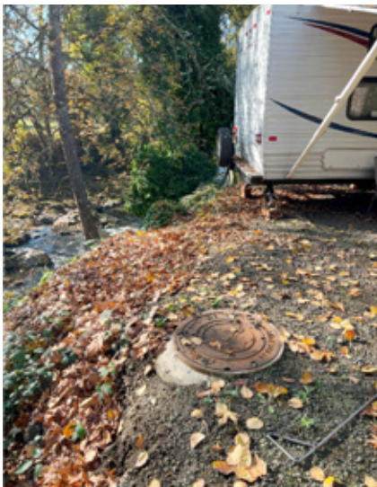
Figure 1. Manhole Along Deer Creek Trunk, Adjacent to Steep Slope
