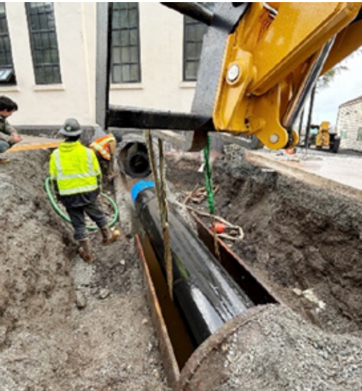
Figure 6. Slipline Access Pit Near SSSC Hatchery
