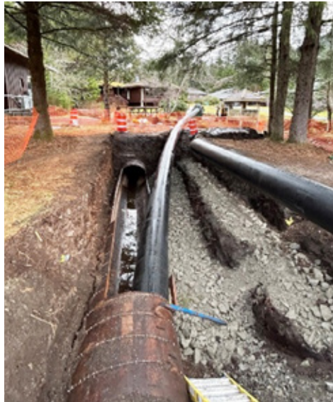
Figure 7. Slipline Access Pit Near Penstock Inlet Near Penstock Inlet air
