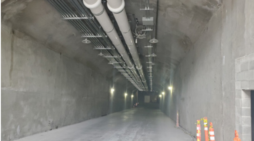
Figure 7: Completed Climate Pledge Arena Tunnel
