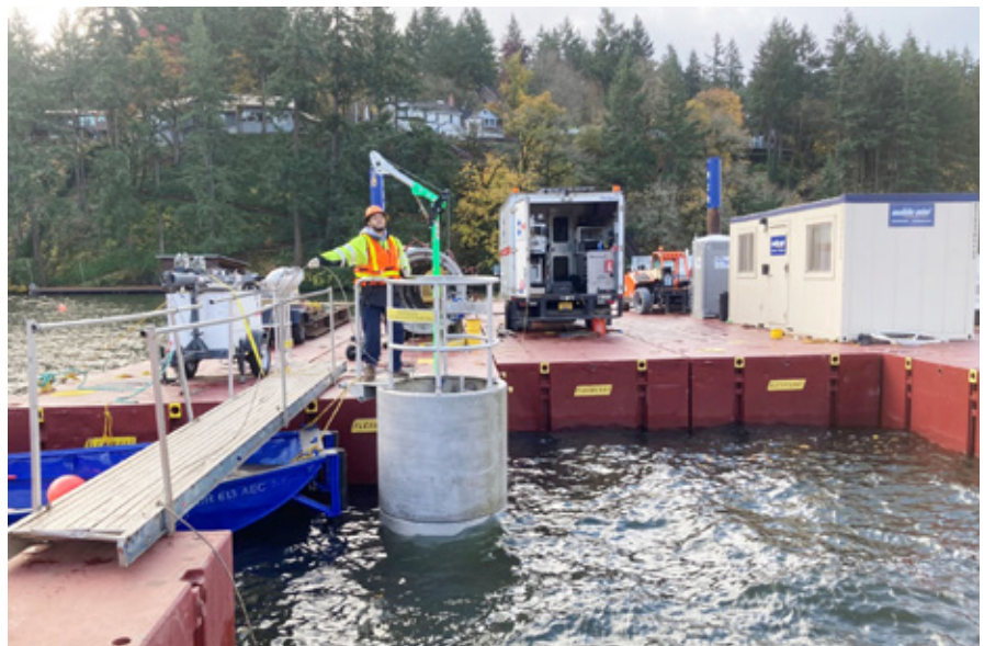
On water inspections were completed in 12 weeks
