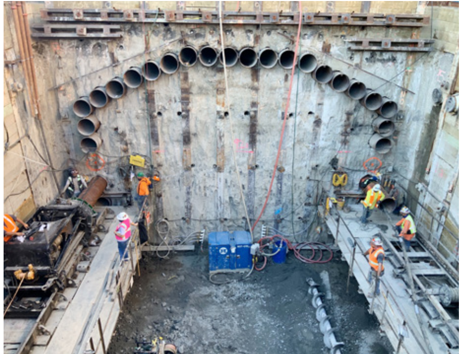
Figure 4: Example of boulders encountered during excavation
