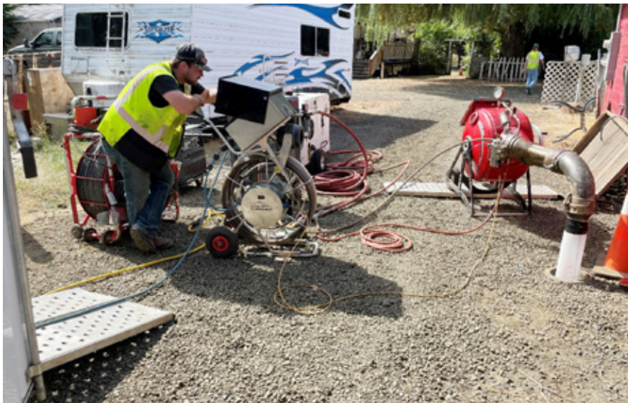
Figure 6. LED lateral lining through existing cleanout
