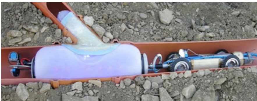
Figure 7. Cosmic Tophat Lateral Connection Liner
