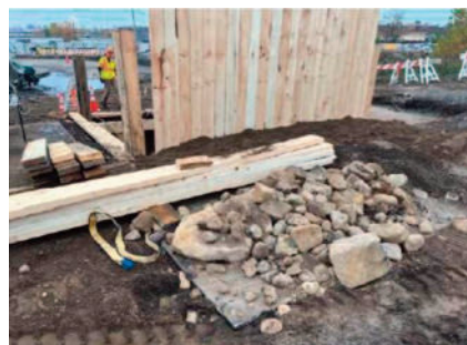
Figure 3. Cobbles and Boulders from Pit Excavation
