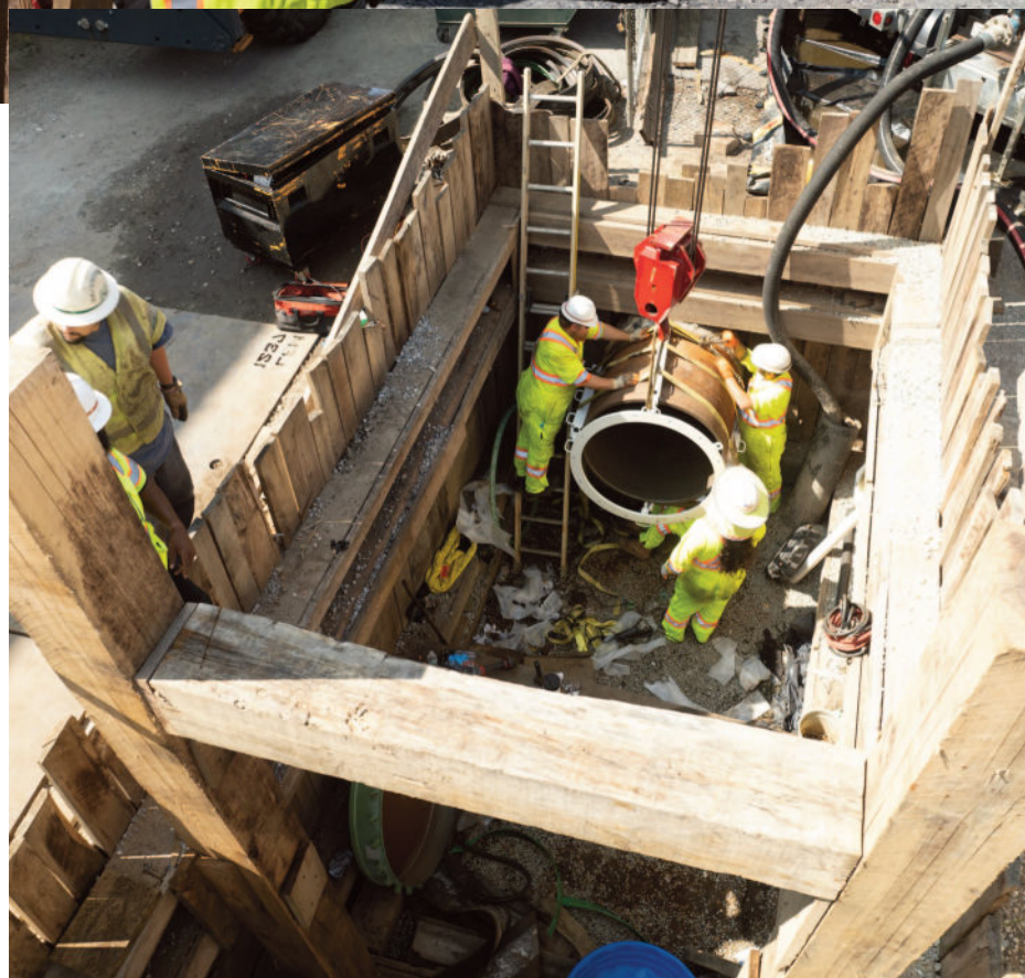
Inside the pit, the 42-inch pipe is being prepared to receive the liner
