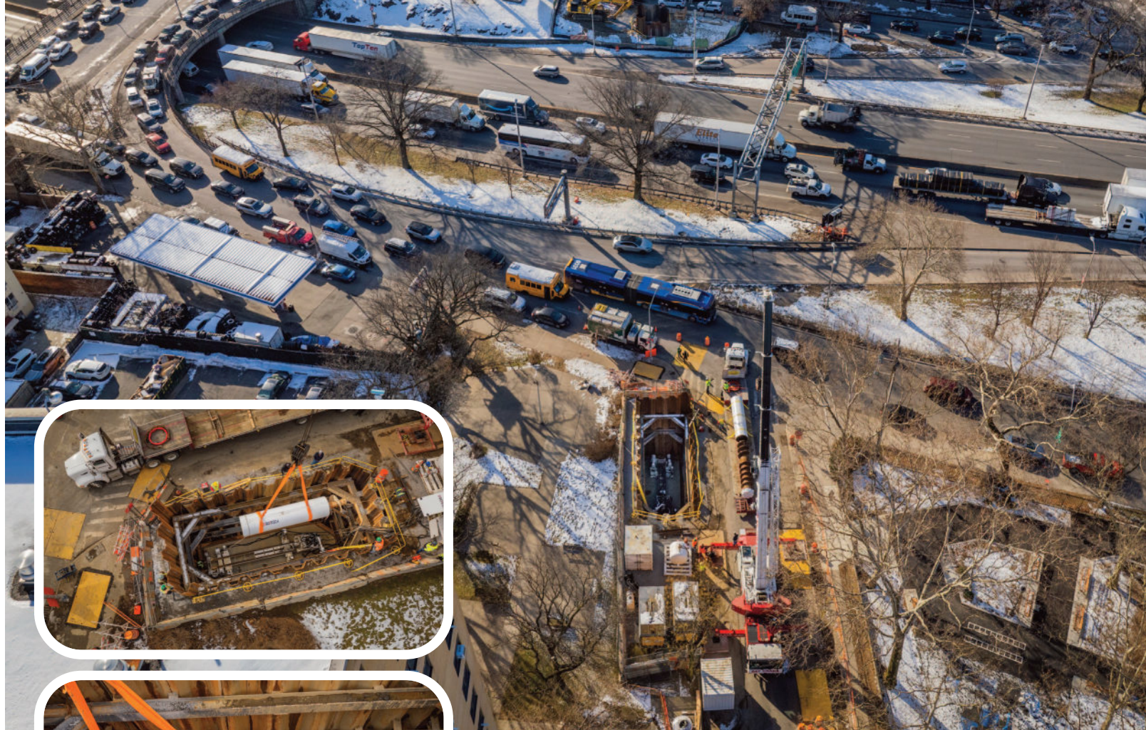
I-95 Cross Bronx Expressway is the most congested corridor in the US. Sending pad 40 feet in length to accommodate both drill and 20-foot casing length segments
