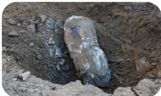
LEFT: Boulders as large as 10 feet were excavated and removed from the jacking shafts.
