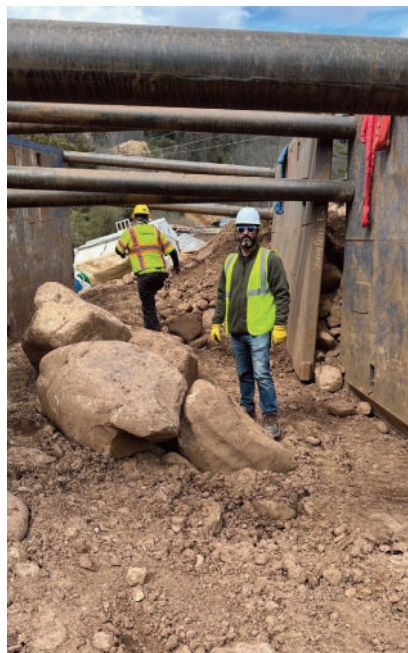
The cobbles and boulders encountered required a search for an effective trenchless method
