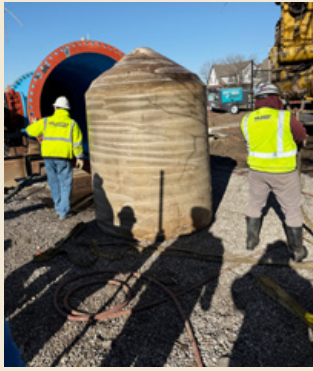
Debris pushed out from the medium density bare pig (left) included 5-gallon drums, an extension cord and grout
