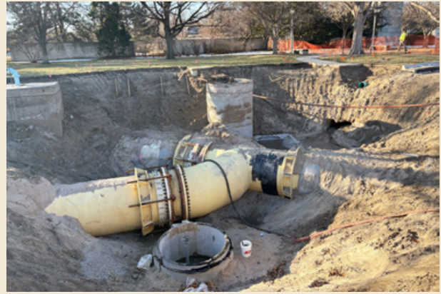
The 90-degree turn through a tee that led to the newly constructed section of pipeline towards the retrieval point
