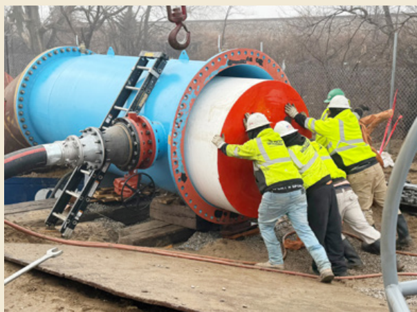
An external pump was used to launch the pig into the pipeline until the point that it was propelled by the system water flow
