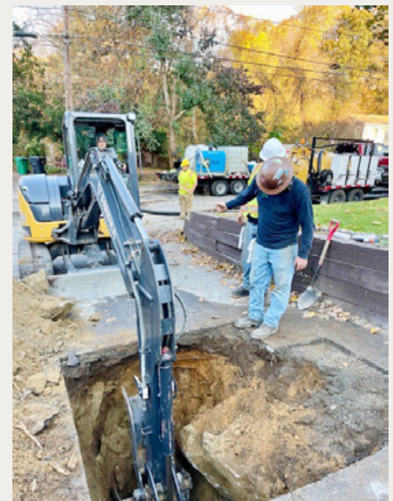
Figure 9. Ground predominantly hard pan with large cobbles, boulders and shale
