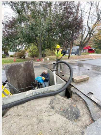
Figure 8. The new HDPE pipe was pulled back to the collector main located at the starting pit
