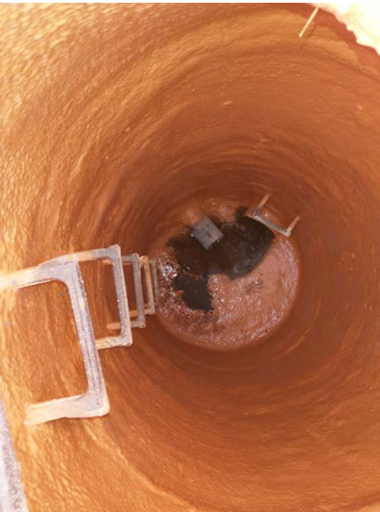
Manhole successfully lined with OBIC products to stop I&I
