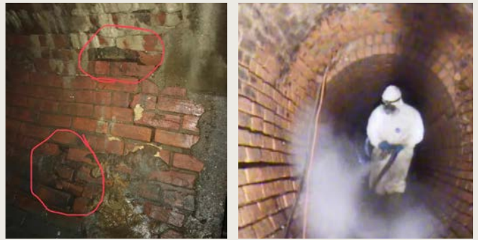
Figure 5: Typical Brick Pipe missing mortar prior to shotcrete of geopolymer
