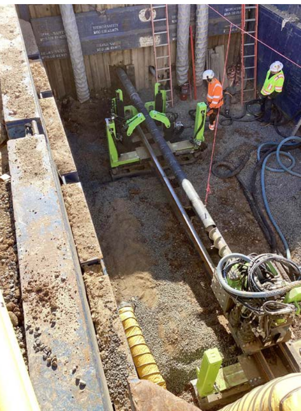
Figure 6. Down the Hole Hammer Machine in Pit
