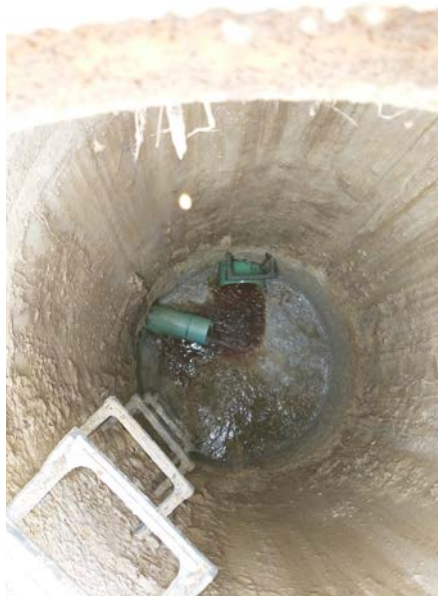
Severe I&I captured in a manhole in the Village of Hamler
