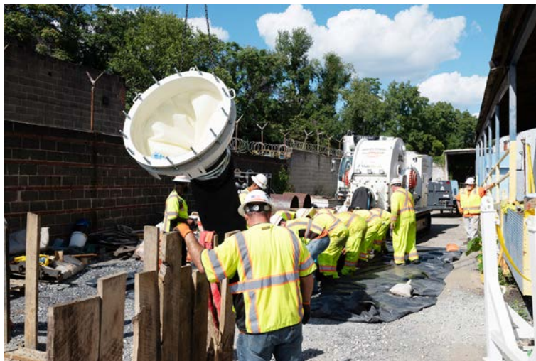
The Starline® CIPL drum, liner and transfer hose moving into the pit for lining
