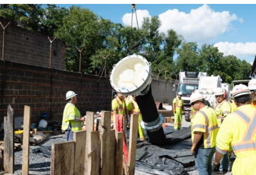
Inside the transfer hose, the liner was pneumatically inverted and moved through the pipeline
