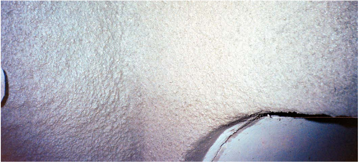
Figure 2: Finished SewperCoat® 2000HS surfaced sprayed 3 inches thick
