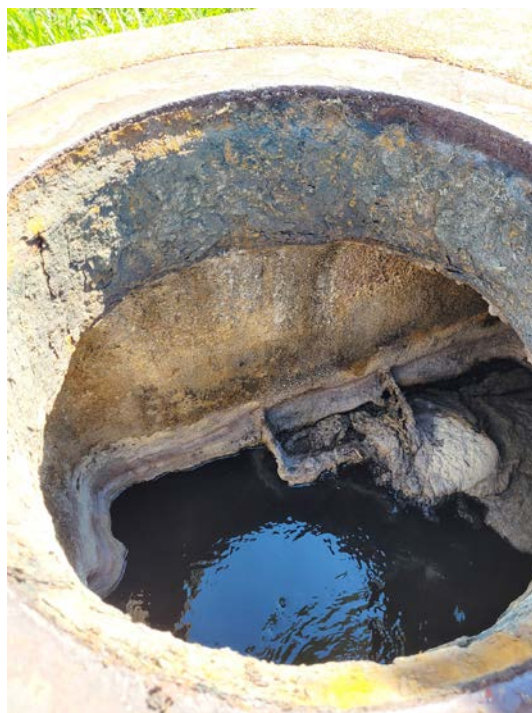
Figure 6: 31-Yr Evaluation - SewperCoat® still hard and corrosion free
