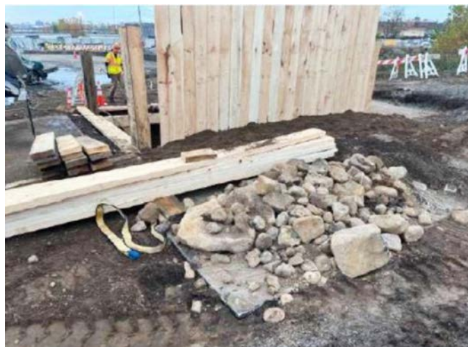
Figure 3. Cobbles and Boulders from Pit Excavation
