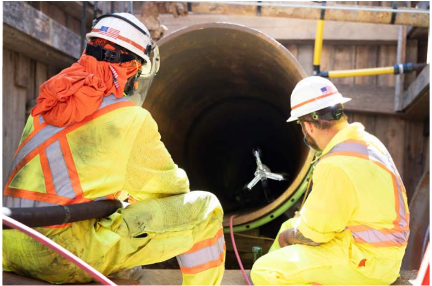
The 42-inch cast iron internal pipe surface was cleaned and prepared using grit and a spin blaster
