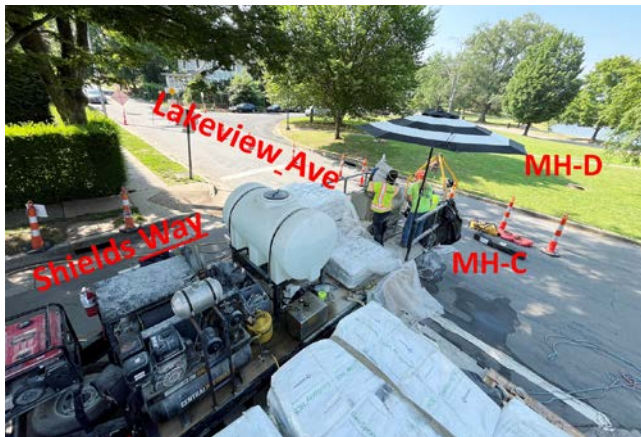
Figure 3. Generator, compressor, water tank, geopolymer pallets and mixer are carried on one flatbed
