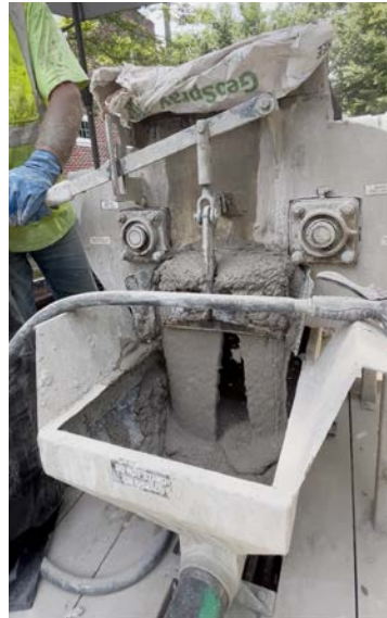
Figure 7. Geopolymer and water blended in mixer, dumped and pumped
