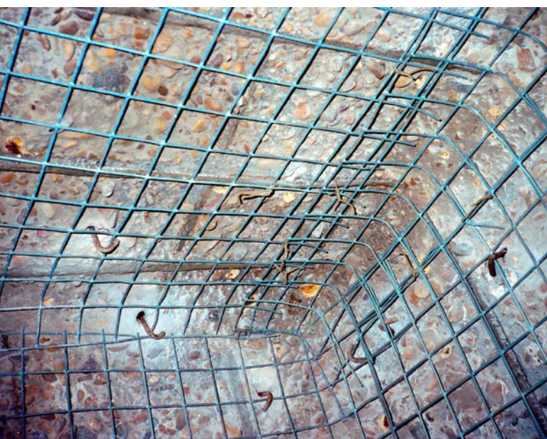
Figure 1: Damaged OPC showing exposed aggregates and prepped with new rebar to begin coating
