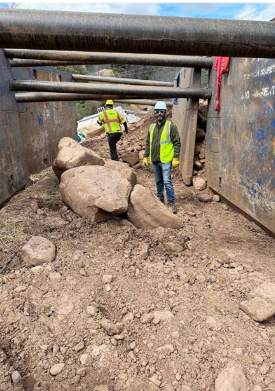
The cobbles and boulders encountered required a search for an effective trenchless method
