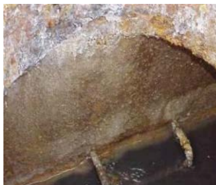
Figure 5: 11-yr evaluation- SewperCoat® continues to perform even as the surrounding iron frame begins to deteriorate
