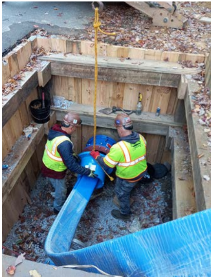
Uniquely engineered liner design accommodates multiple bends
